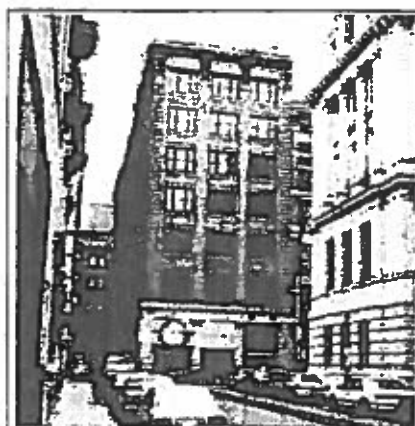
Fig. 29f Typical downtown loft building
